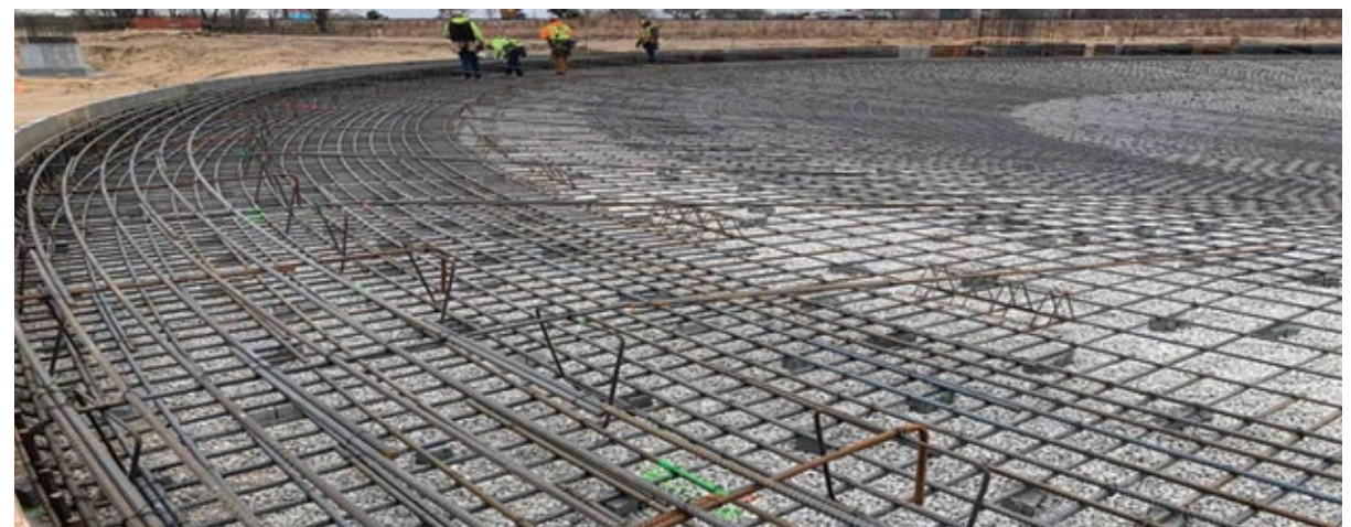
Top: Aerial view of the site, looking east. Bottom left: Construction work at the solids contact clarifiers. Bottom center: Interior concrete construction and pipe installation at the filter building. Bottom right: Reinforcing bar installation at the solids contact clarifiers.
